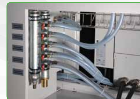
Central water supply
